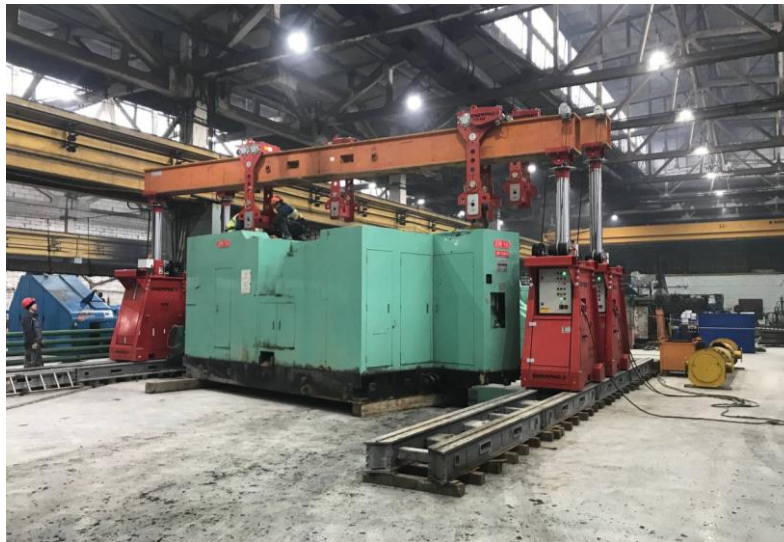
Moving and mounting of pressing equipment LLC Oryol steel rolling plant, Oryol, 2022
