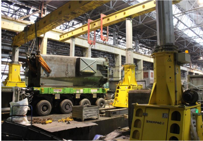
Moving and mounting of pressing equipment LLC Oryol steel rolling plant, Oryol, 2022
